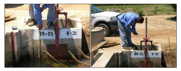
Figure 2. District staff measuring water at a modified constant-head orifice turnout in an Alta Irrigation District canal
